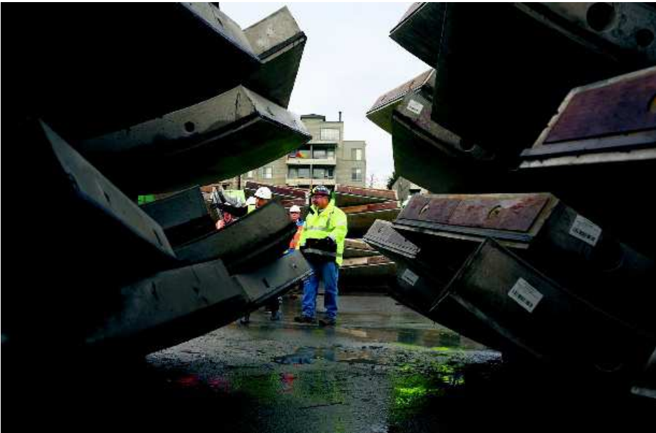
Engineer Jim Salley explains the tunnel segments, six of which fit together to form one five-foot long ring of tunnel. Seattle’s new stretch of rail lines will travel across Capitol Hill and to the University District.
